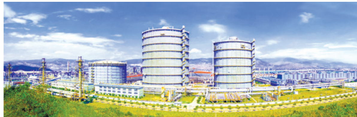
Coal gas storage and distribution station
