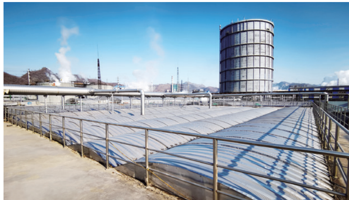
Beiyang coking phenol and cyanide containing wastewater odor treatment facilities
