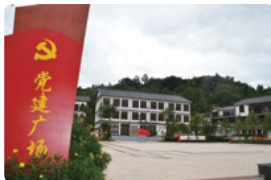
↑ Gaoguan Village Party Building Office
