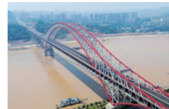
The longest arch bridge in the world-Chaotianmen Yangtze River Bridge in Chongqing (Ansteel Group high-performance bridge steel Q420qD)
