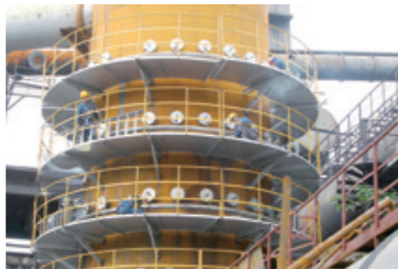
New dust-removal equipments of Pangang Steel and Vanadium was almost completed
