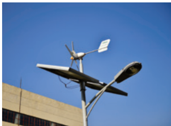
LED Energy-saving Lamps Installed in Resource Utilization Center of Pansteel Group Steel Vanadium & Titanium Co., Ltd.
