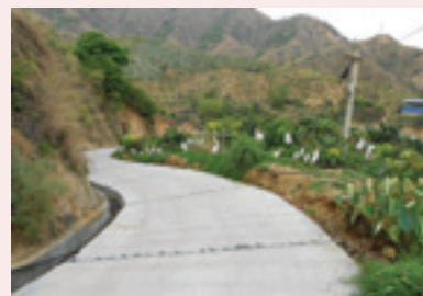
Roads Build by Pansteel for Impoverished Villages
