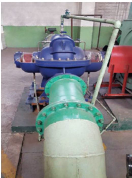
Cold-rolled Recycling Water Pumps of Pansteel Group Steel Vanadium & Titanium Co., Ltd.
