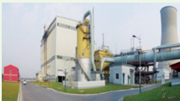
The CCPP Unit of Anshan Iron and Steel Second Power Plant
