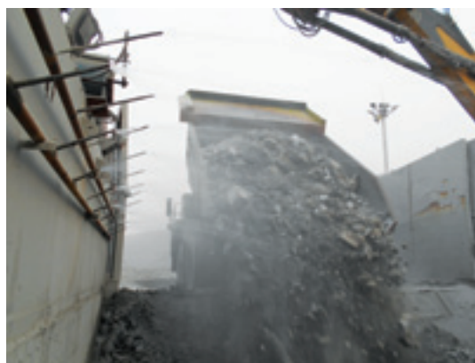
Water Removing Dust of the Crushing Station
