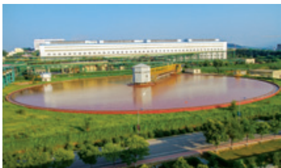
The Largest Domestic Tailings Settling System with a Diameter of 140 Meters
