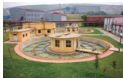
Wastewater Recycling and Reclaiming System
