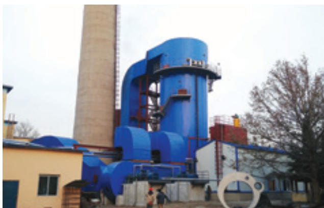
Fume Desulfurization for Boilers of East Anshan Sintering Plant
