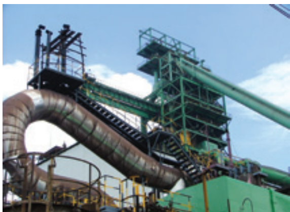
Pansteel TRT Waste Heat Power Generation
