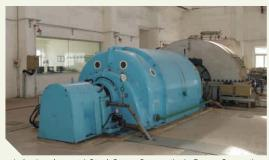
▲ Anshan Iron and Steel Group Corporation's Power Generating Units Using Waste Heat from Sintering Machines.
